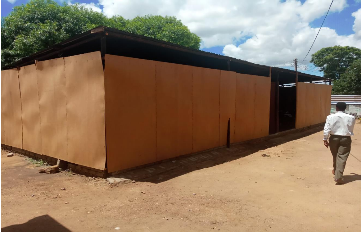
Picture 2: One of the Classroom Facility at Vision Academy made up of hard boards
